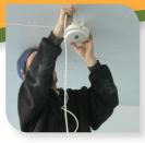
By comparison, sound masking components are small and the installation process tidy. They can typically be installed without conduit in most jurisdictions. The work can be handled discretely after hours or with only minor disruption to occupants during regular hours. There are few requirements for power tools, making the work relatively quiet, and unless the ceiling is unusually high, only ladders are needed to gain access.
